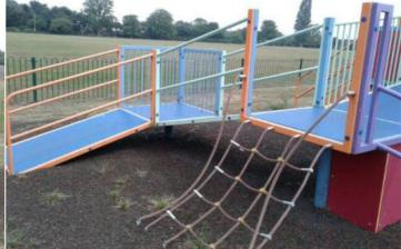
**Finding:** There is an opening in the barriers exceeding the width allowed (500mm) in BS EN 1176, this is a low risk failure and no remedial action is required
