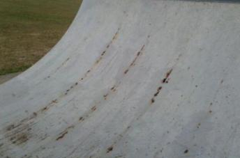
**Finding:** The riding surface of the ramp is severely damaged- The damage on the surface of the ramps suggests that the metal riding surface is deteriorating we recommend an internal inspection of the item is carried to ascertain the structural stability of the item
