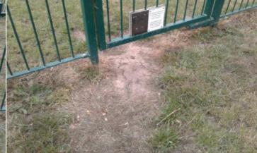
Finding: The surface has eroded in some areas Action: Reinstate the surface
