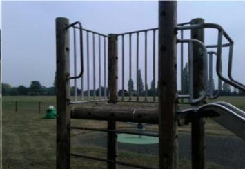
**Finding:** There is an opening in the barriers exceeding the width allowed (500mm) in BS EN 1176, and no guardrail has been provided; this is a low risk failure and no remedial action is required
