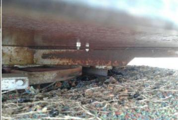
**Finding:** The underside of the rotating platform shall be smooth for the first 500mm towards the axis to comply with the requirements of BS EN 1176 Part 5
