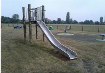
**Finding:** The timber edging forms a hard object within the falling space of the equipment in contravention of the requirements of BS EN 1176 Part 1
