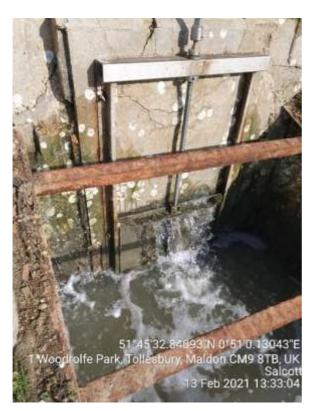
This image shows the view of the Sluice Gate with water leaking which is due to the flap not working correctly.
