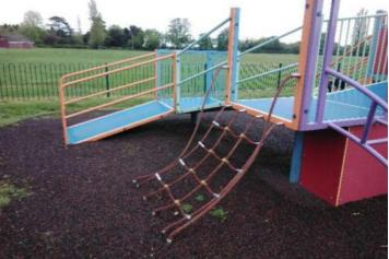
Finding: The unit is easily accessible and should have the Action: Monitor - No remedial work recommended appropriate barriers installed to meet the requirements of BS EN 1176 Part 1 as the height of the unit exceeds 600mm
