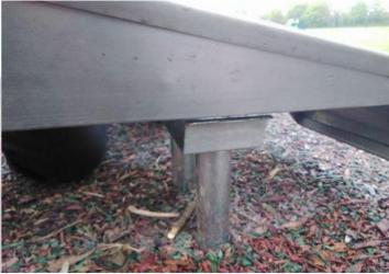
Finding: The weld(s) on the slide run out have failed
