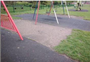
Action: Reinstate the surface Finding: The surface has eroded in some areas
