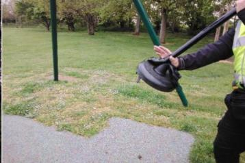
Action: Adjust the cable stop position to ensure the Finding: The seat is less than 2.0 metres from the post when extended at 45 degrees at the end of the area of travel minimum distance is maintained and does not meet the requirements of BS EN 1176 Part 4
