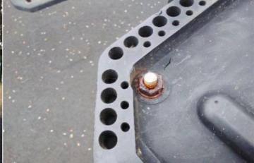
Finding: The fixings have corroded excessively
