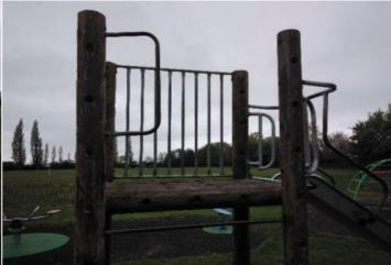
**Finding:** There is an opening in the barriers exceeding the width allowed (500mm) in BS EN 1176, and no guardrail has been provided; this is a low risk failure and no remedial action is required
