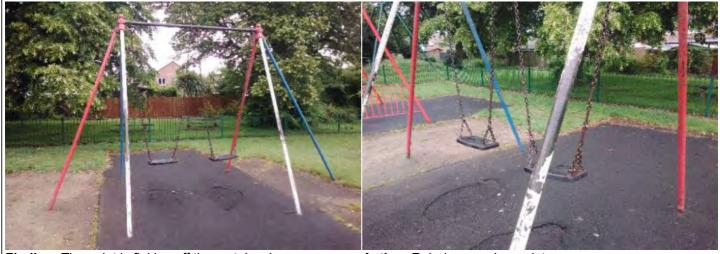
Finding: The paint is flaking off the metalwork
