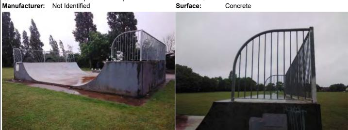
Finding: The height of the barrier is less than 1200mm and Action: Monitor - No remedial work recommended fails the requirements of BS EN 14974
