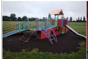
Finding: The item fails to meet the requirements of BS EN Action: Monitor - No remedial work recommended 1176 Part 1 4.2.7.2 head and neck entrapment in the barriers and/or steps
