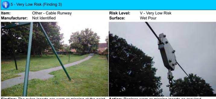
**Finding:** The nylon inserts are worn or missing at the point **Action:** Replace worn or missing inserts as required the cable enters the traveller
