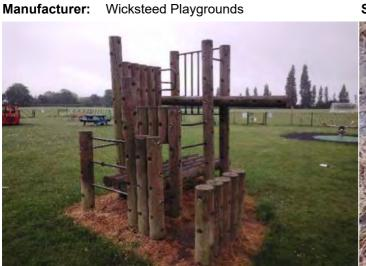
Finding: There is some strimmer / machinery damage apparent on the posts, this can penetrate the preservative applied to the timber and accelerate the rotting process
