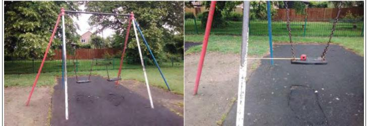
**Finding:** The seats are too close to the frame as defined in **Action:** Monitor - No remedial work recommended BS EN 1176 Part 2; this is a low risk failure and no remedial action is required
