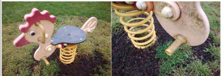
**Finding:** The end of handgrips and/or footrests have a cross **Action:** Monitor - No remedial work recommended section of less than 15cm2 and fail to meet the requirements of BS EN 1176 Part 6
