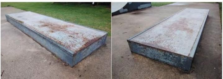
Finding: The paintwork on this item has been damaged or Action: Treat any rusting components and repaint worn exposing the metal underneath which is rusting
