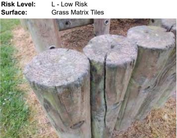
Finding: The timber has a number of splits/shakes or air Action: Monitor to ensure the splits do not cross through cracks and this may affect the stability or allow water ingress fixing points of the structure and/or cause any instability which will accelerate the rotting process
