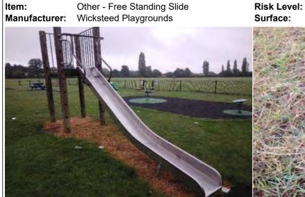
Finding: There is some strimmer / machinery damage apparent on the posts, this can penetrate the preservative applied to the timber and accelerate the rotting process
