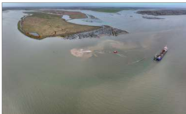
Figure 6. Discharging by pipeline at the start of the ebb at Old Hall on 3 January 2022 @ 12:54 pm (the day before readings were collected).
