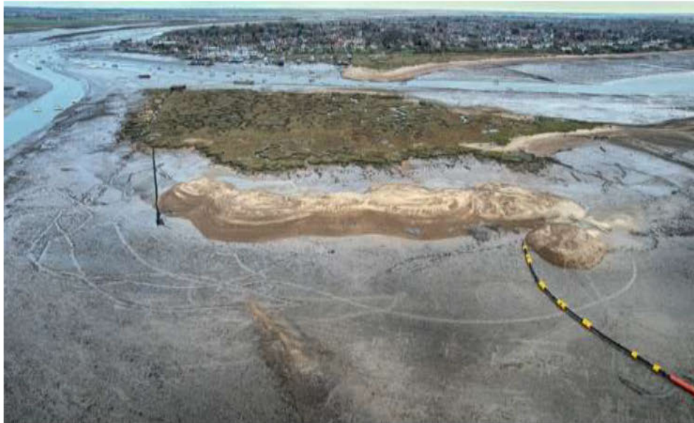
Figure 8. Cobmarsh Island after delivery of the 6th hopper load. The pipeline remains in place at low tide to be reconnected to the dredger when it returns on the next tide; a further 31 loads were delivered. Line of retention fencing on the west side of the recharge (see Section 6). View north: Mersea Island in the background and Mersea Fleet to the west.
