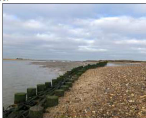
Figure 26. Structure of the retaining fence, northern end of Cobmarsh Island (Mark Dixon).
