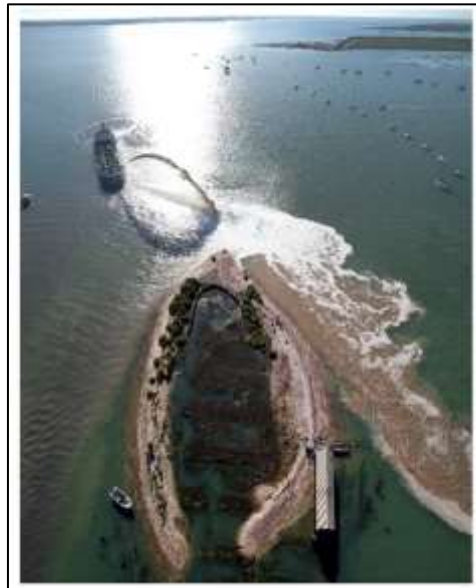
Figure 4. Sediment plume in Thorn Fleet drifting north-westward during rainbow delivery as dredger discharges 47 minutes before the ebb.
