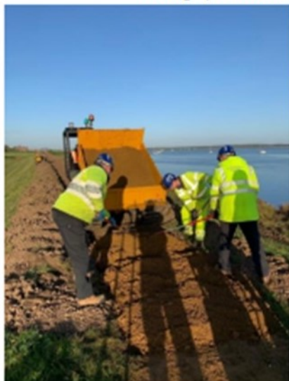
Photograph above: Operatives compacting the Carstone
