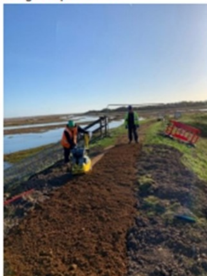
Photograph above: Importing Carstone to the crest
